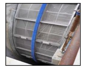
Figure 4-56: Intake Bar Screen
