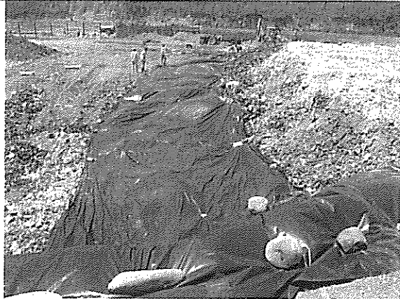
Figure 3. Ongoing Landfilling activity
